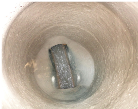
Manhole After Rehabilitation
